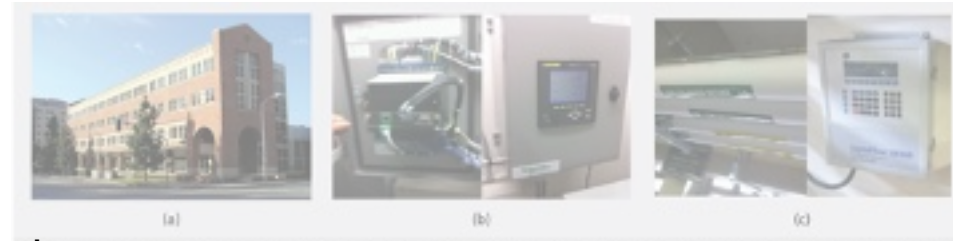
UCLA Strathmore building monitoring system deployment: a) monitored building; b) electrical demand monitor; c) water flow meter.
